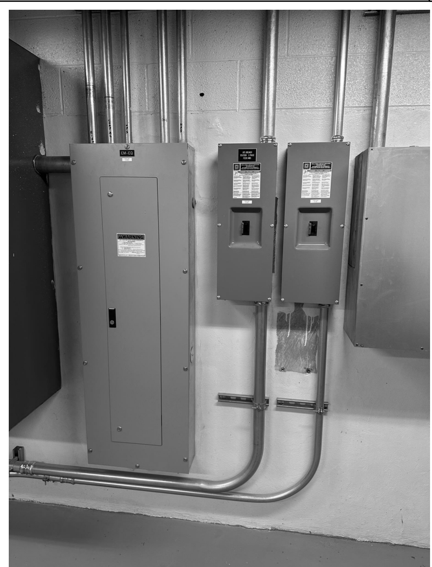
2 E101 EXISTING PANEL "EM-EQ" SCALE: NTS
